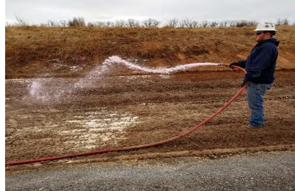
Application of EnviroClean® Treatment over Impacted Area
