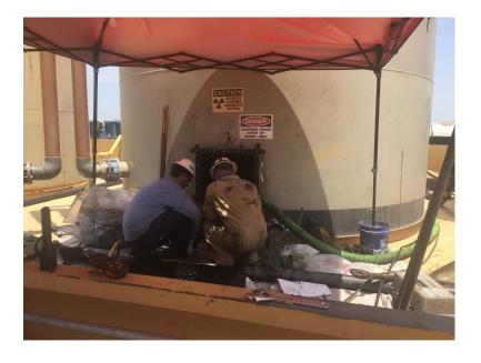
Once the tanks were cleaned, a Ludlum Model # 3 meter was utilized to determine if any NORM remained within the tanks.
