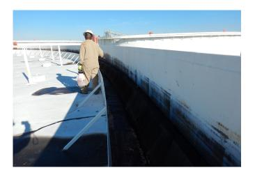
Crews performed a visual inspection to ensure all remaining liquids and sludges within the tanks had been removed prior to beginning power washing activities.
